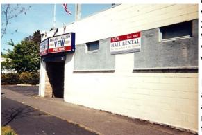
of each window. When we installed the paneling in the main hall we insulated and covered the windows on the inside. Finally, in 2003 we hired a mason to take out the windows and fill the spaces with concrete blocks to match the existing. If you look closely when you visit the hall you can see the new blocks contrasting with the old.
